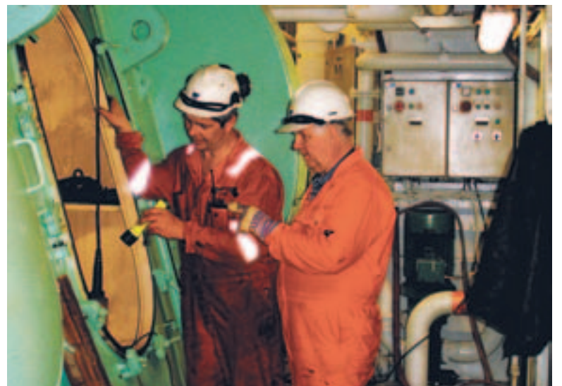
Visual inspection confirms the excellent overall condition of the running gear.
